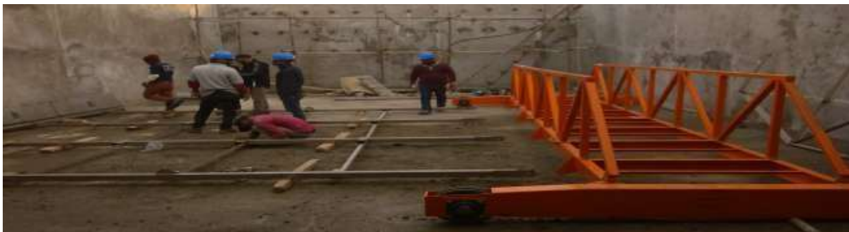
Design and Engineering of 1.4 MGD Water Treatment in Filtration plant, Islamabad, Pakistan 2019
