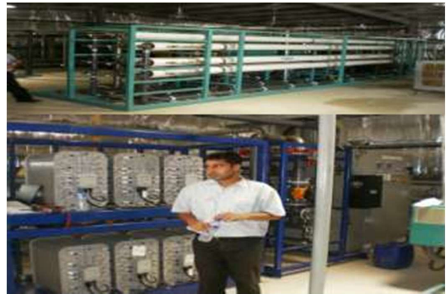
Naduro Sugar Power plant 47 m3/hr RO + CEDI 2011
