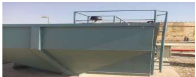
Package Plant Sewage Treatment Plant, Karachi 2014 Capacity 5000 GPD 2014
