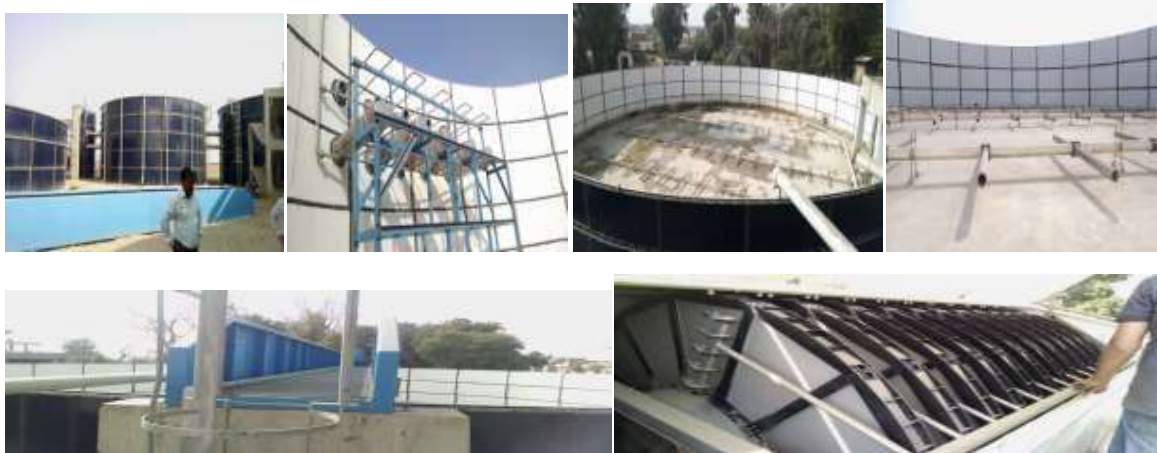
Installation of 6 MGD MBBR Sewage Treatment Plant Sindh , Pakistan 2016
