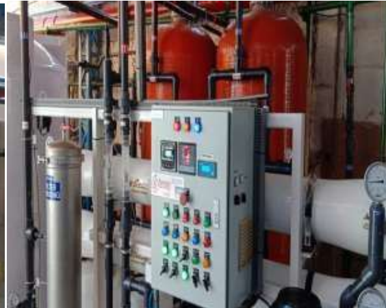
ICI Pakistan RO plant with hot water sanitizable membrane 2020
